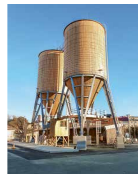
Two log silos in Vienna, each with a capacity of 500 m 3 .
