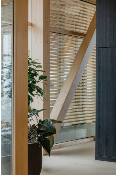
View from the inside, looking towards the southwest facade made of spruce lamellas, inspired by the image of the boards stacked to dry in the neighbouring sawmill Photo credit: Jan Thoma | Blumer Lehmann
