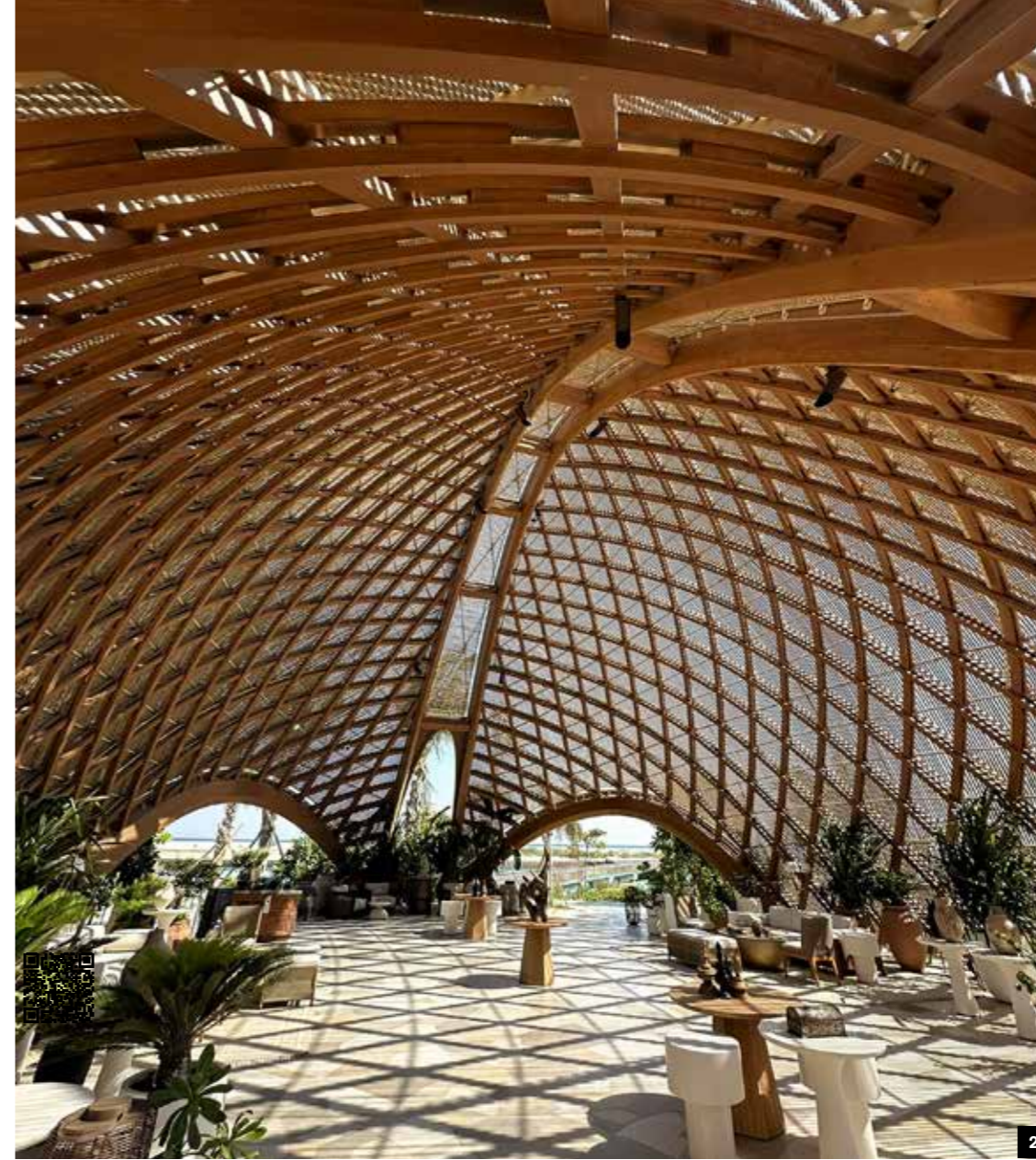
1+3 Kengo Kuma's design for the water villas, with their spiral shape and panoramic views, is inspired by sea corals. 2+4 The Free Form roof structures of the Nujuma Ritz-Carlton Reserve flow organically, expressing the elegance of complex timber geometry.
