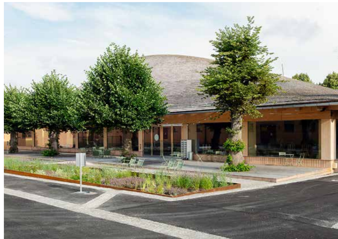
The unsupported Free Form roof made of laminated veneer lumber and arranged as a visible lattice shell spans an area of 25 x 48 m.
