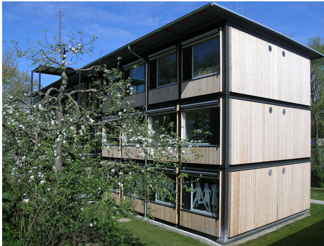
Temporary school building: the temporary and modular buildings that Blumer Lehman produces can be prefabricated in the factory, resulting in short construction site times, which is a huge advantage when building in urban areas.
