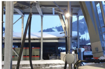
Mobile electric conveyor system for returning salt from the gritting silo in Airolo
