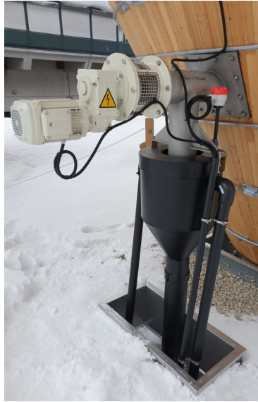
Brine generator with salt dissolving system and storage tank with mixing station
