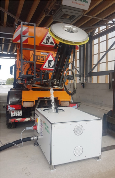
Modular silo facility for gritting materials in Fribourg
