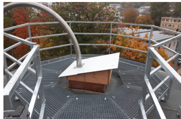
Filling hopper with loading bellows
