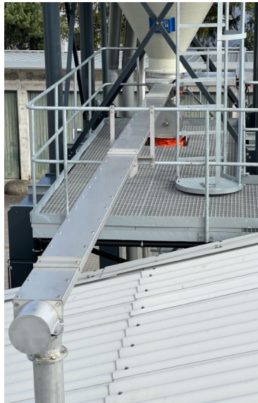
100m 3 GRP silo with brine generator and 50m 3 GRP storage tank
