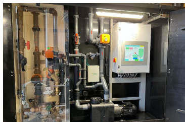
Interior view of brine generator with integrated blowdown system for brine recovery
