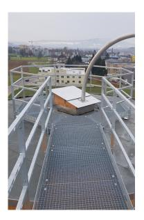
Silo funnel with height-adjustable windsock, unbalance vibrator and knocker made of oak wood
