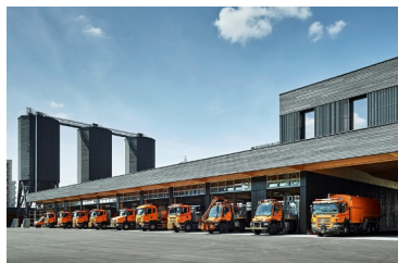
three dodecagonal timber silos with a volume of 900m 3 each in Bern Wankdorf
