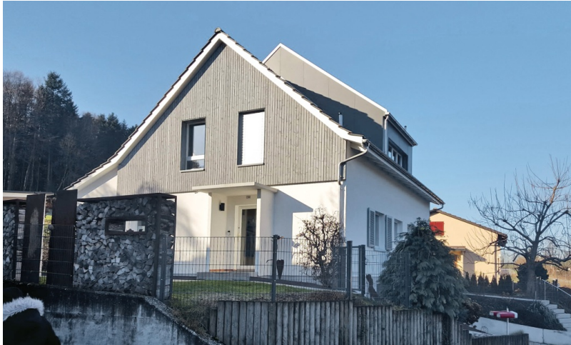
View of the additional storey and roof extension.
