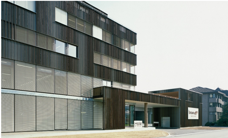
Entrance area of office building
