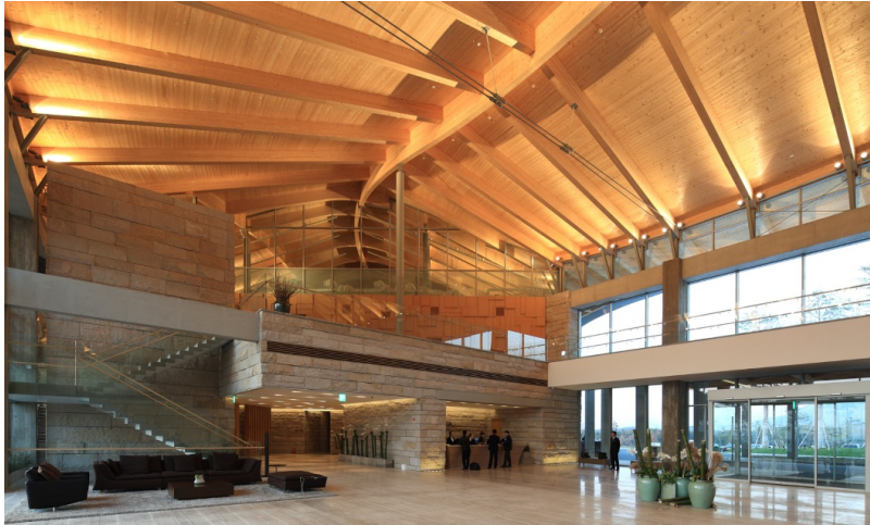
Sweeping, leaf-shaped roof construction
