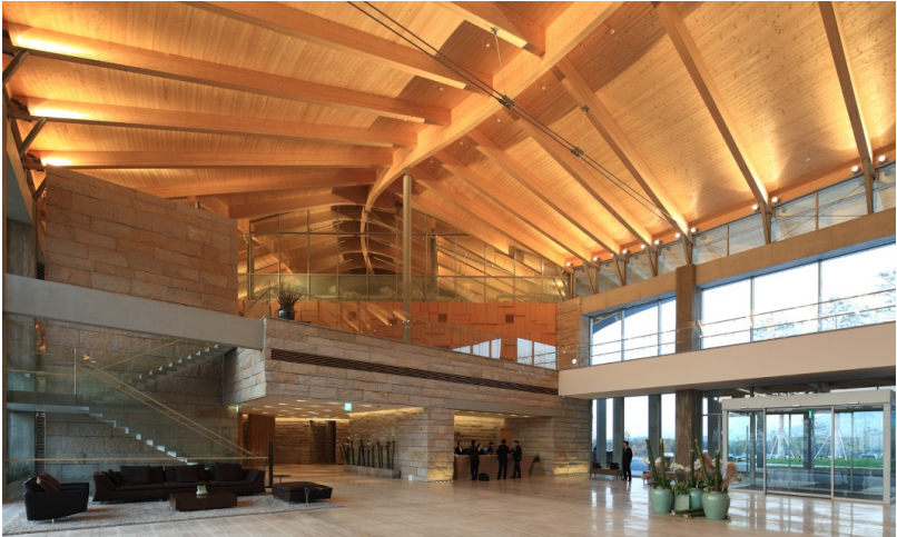
Sweeping, leaf-shaped roof construction
