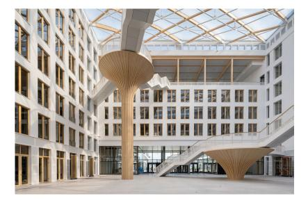
The cladding for the steel supports is formed from spruce timber strips.
