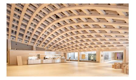
The unsupported Free Form roof made of laminated veneer lumber and arranged as a visible lattice shell spans an area of 25 x 48 metres.
