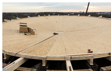
Detailed view of the roof construction during construction work
