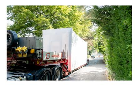
The individual timber modules were prefabricated at our factory in Gossau and then transported by low loader to the construction site.
