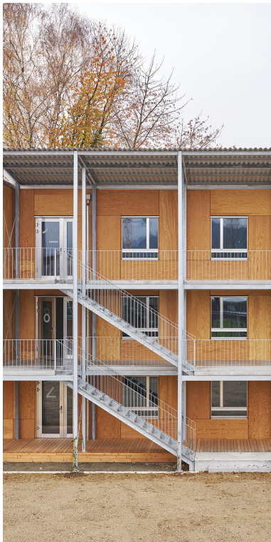
Staircase connecting the three storeys
