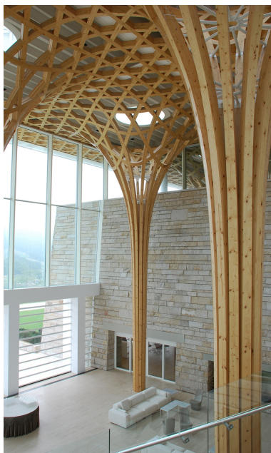
Decorative effect of the support structure
