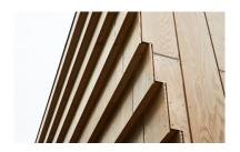
The wooden façade with conventional cladding corresponds to the traditional construction in the area.
