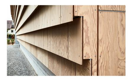
The façade made of wooden panels provides natural ventilation of the warehouse.
