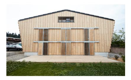
The vertically laid wooden façade panels offer protection from wind and rain.
