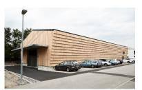
The new building in timber construction fulfils the two central requirements: column-free warehouse and the possibility of placing high-bay racks over the entire storage area.
