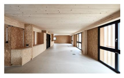
The interior of the warehouse also consists of timber left as raw as possible.
