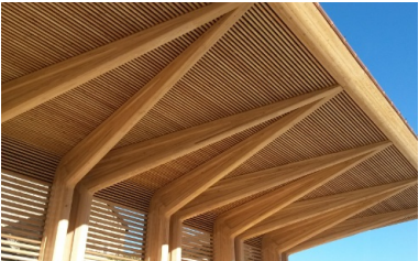
Close-up of the roof construction
