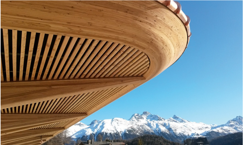
Unique roof construction in larch
