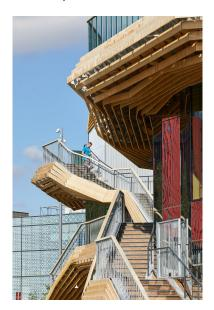
The external steel stairway, clad in timber, provides visitors with access to the roof garden.
