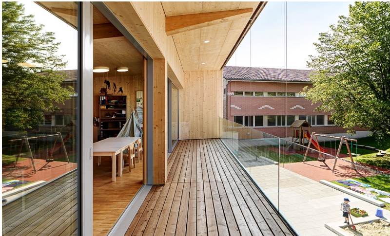
An airy classroom in the new projecting structure on the top floor.
