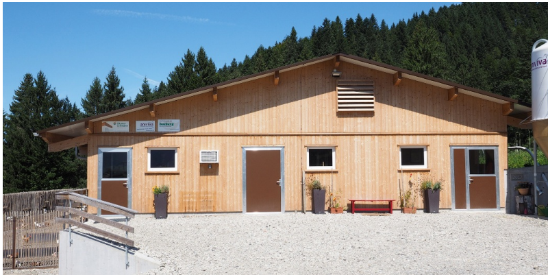
Front side with spruce/pine cladding
