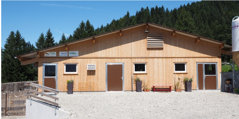
Front side with spruce/pine cladding
