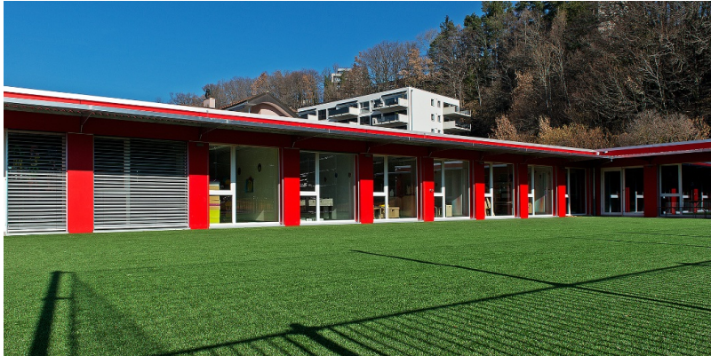
Single-storey modular construction
