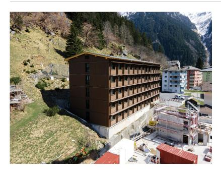
The Dammastock modular timber structure is the largest of the three buildings that make up the Breiti residential complex.
