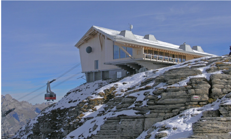
South-west view of the mountain restaurant
