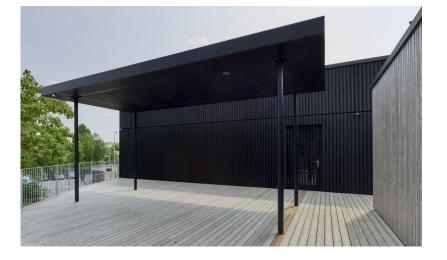
The wooden modules and elements were prefabricated in our production hall in Grossenlüder.
