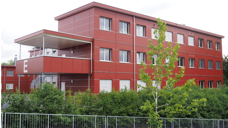
Accentuated colour scheme on the facade
