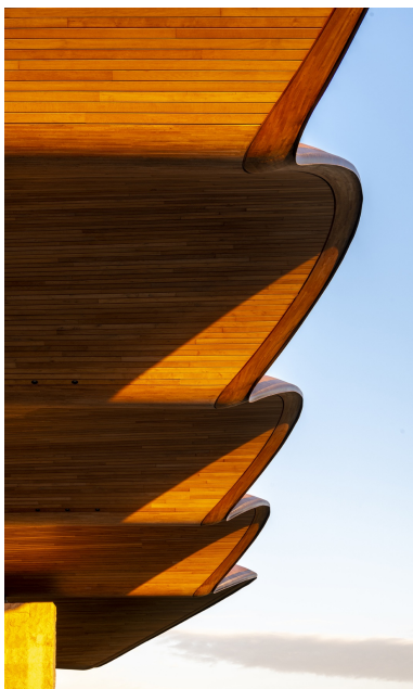
Impressive roof construction in oak
