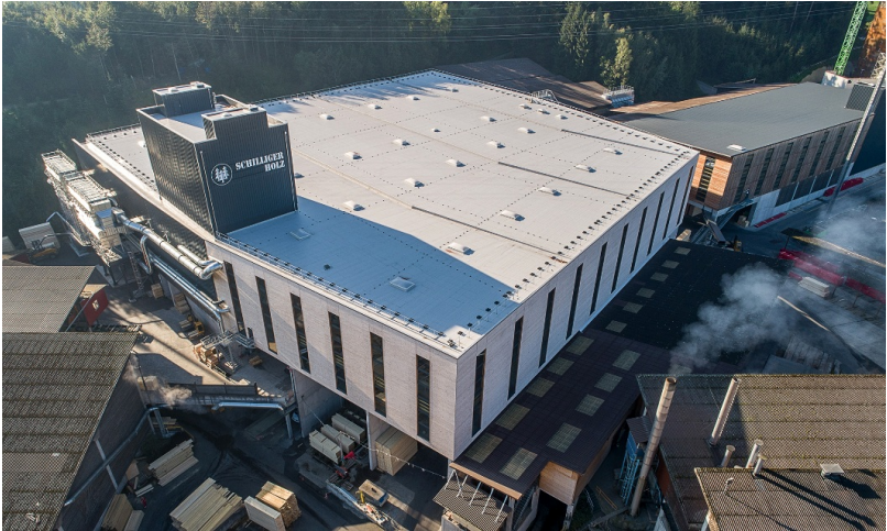
An impressive new building in a prefabricated design.
