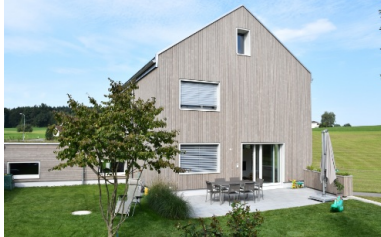
Exterior view of the front
