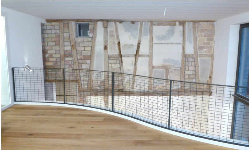
Renovating the old masonry
