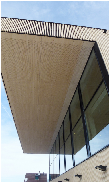
View of the soffit
