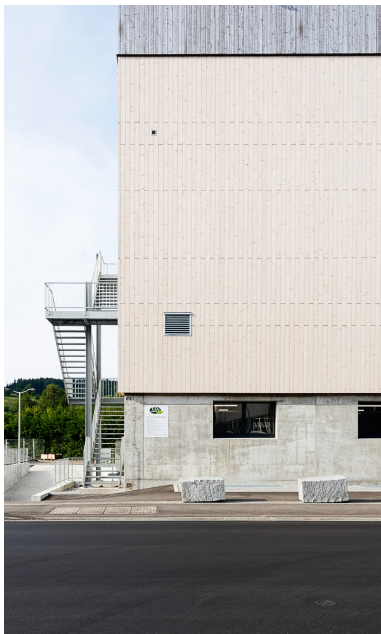
Visibly different: pre-greied wood in the upper section and UV-treated wood below.
