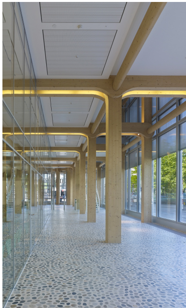
Exposed support structure inside the building
