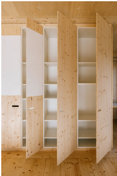
The interior features practical fittings and is made of timber.
