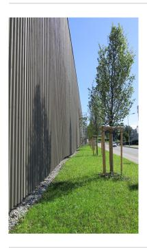
The timber facade made with pregreyed Douglas fir is part of the overall renovation concept to Minergie standard.
