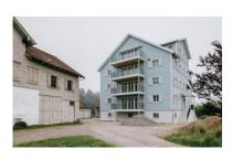
The facade consists of eternit shingles, in keeping with the parameters of the townscape.
