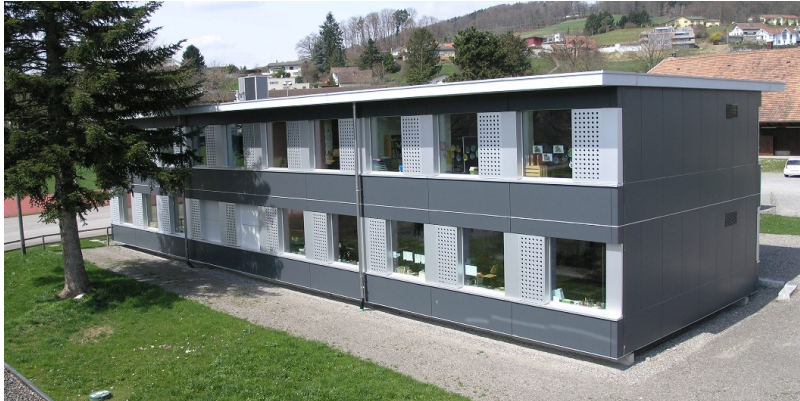
Two-storey Modular-X modular construction
